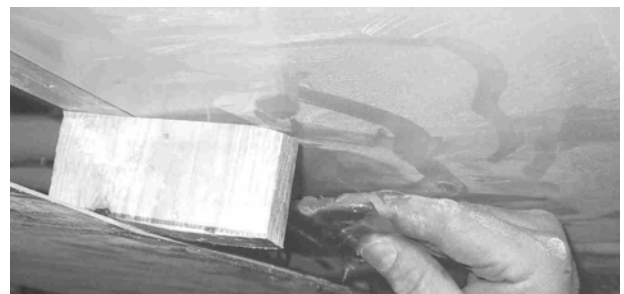
Figure 18: Bonding the Belly Seam Joggle
