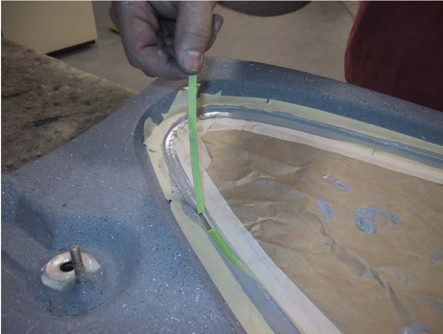
Figure C: Pulling the #2 1/4" masking tape from the window after bonding to the door.
