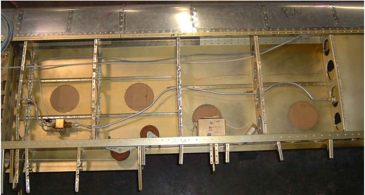
Figure 112: Fuel line routing from the pump to the aux tank. (RH shown)
