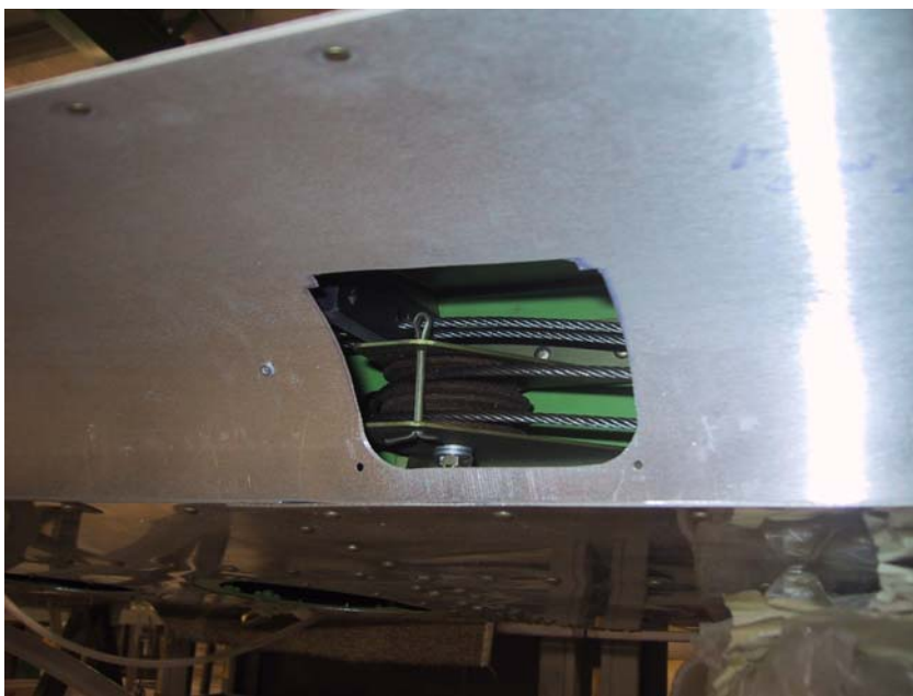
Figure G: Inspection access to pulleys at BL 69.
